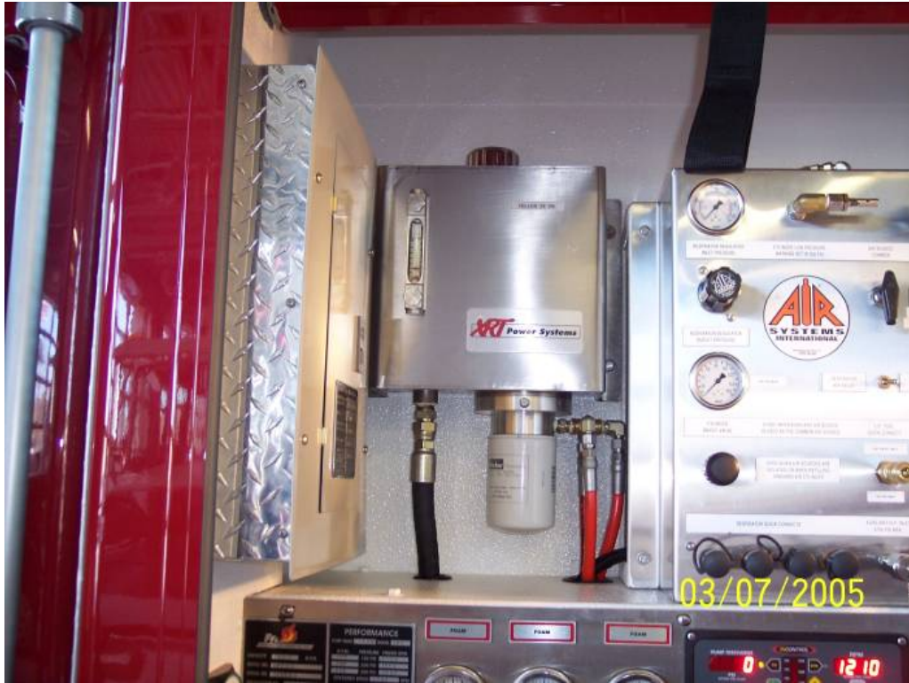
Photo 1 - Oil Reservoir Tank
