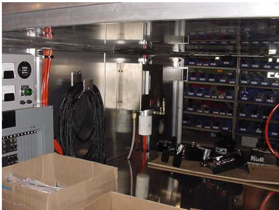
Oil Reservoir Tank (Photo 2)
